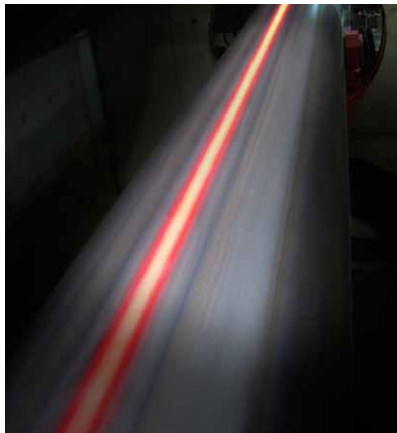
Orbital movement of the coils on this EFD Induction normalizing system means accurate tracking of the weld seam. Normalizing is essential for pipes used in the oil and gas industries.
